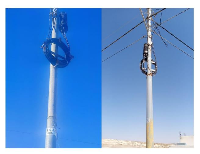
**Cross - Aerial Cable Storage Configuration for Angled Cables**
